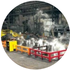
Nucor Utah USA. Mill upgrades.
