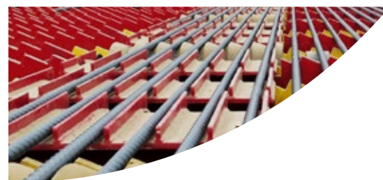
FINISHING END AREAS
